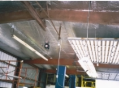
Completed Ceiling Water Management Building
