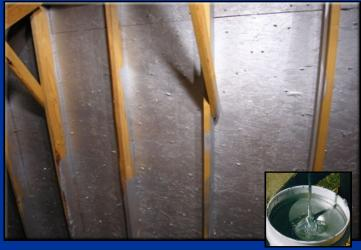
Spray-Applied Interior Radiation Control Coating (IRCC)
