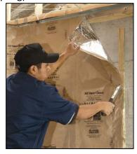
Internal Reflective Air Spaces: Multi-layer reflective insulation requires air spaces between the reflective layers to function at the optimum R-value.
