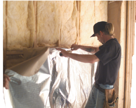
Horizontal application using 54" FSK Shield™ over unfaced batts
