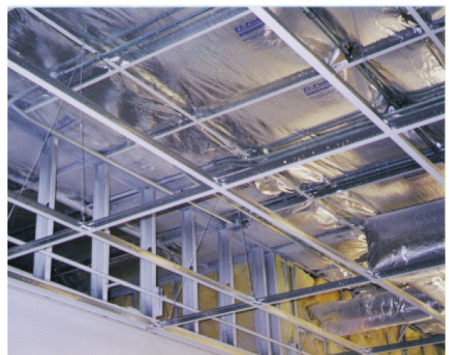
FSK Shield™ adds an R-4.5 to an exposed roof or ceiling application
