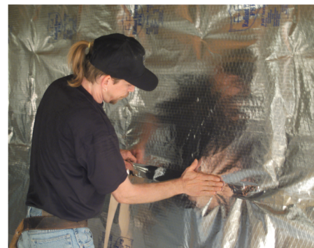
Continuous Class A barrier - less seams than foil-faced batts
