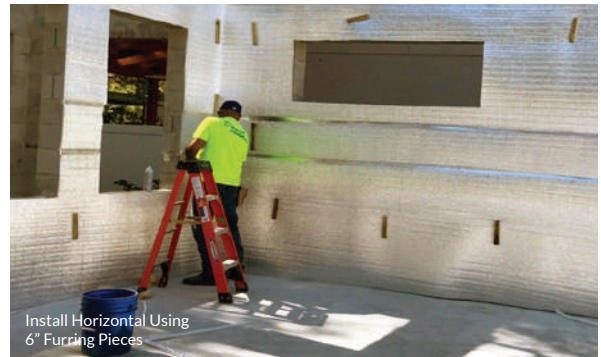
Install Horizontal Using Mechanical Fasteners
